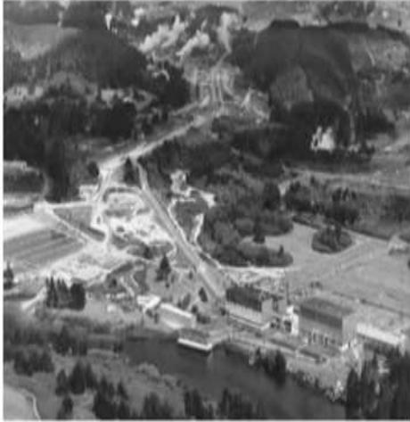
Figure 15.9 The Wairakei geothermal power station in New Zealand. Well-heads are at top of photo; condensed steam is discharged into the Waikato River at bottom. [Photo by courtesy of Contact Energy, New Zealand.]
